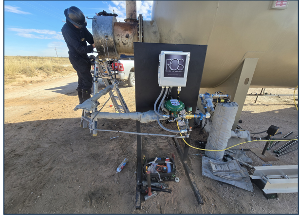
QUICK-CONNECT INSTALL DAY — STAND SET, GAS TRAIN CONNECTED, BURNER WORK IN PROGRESS
