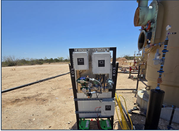
SOLAR + DUAL-BATTERY QUICK-CONNECT UNIT RUNNING A TREATER ON A PAD WITH NO POWER
